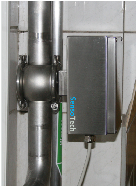
LiquiSonic® Plato application at the wort cooler
